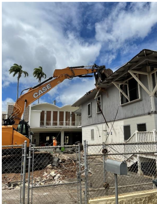
Removing the minister’s residence roof
